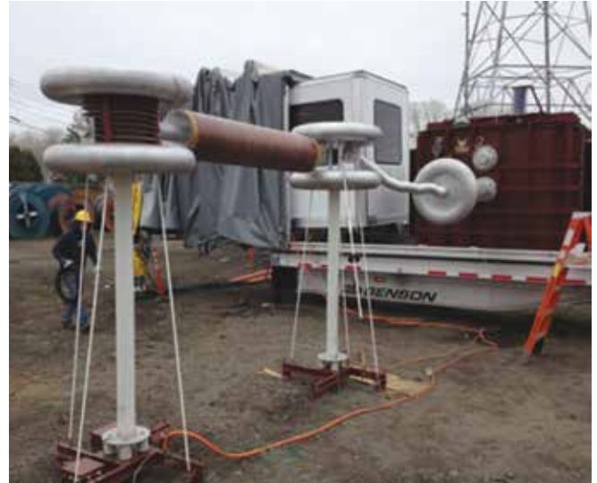
Dielectric testing 138 KV class transmission cable in Long Island, NY.
