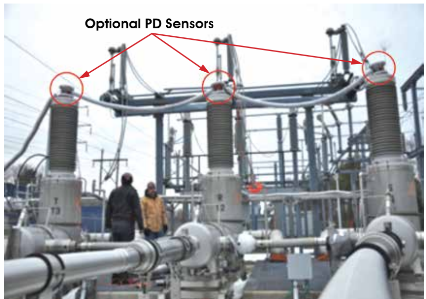
Optional Partial Discharge measurement setup.
