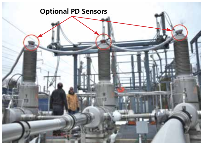
Optional Partial Discharge measurement setup.
